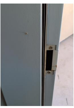
Remote Access Control – Based on field confirmation, devces can be installed. We would recommend that they be installed with a combination of local card reader control with card reader disabled at night and door control shifted to Central Contrl to eliminate the the temptation for youth to try to get the staff access card when staffing is reduced. Further impacts that would have to be resolved is the addition of input/output devices in the head
